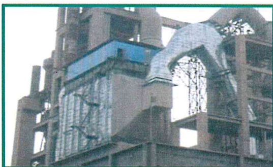
Replaced L-1 C line ESP by Baghouse
