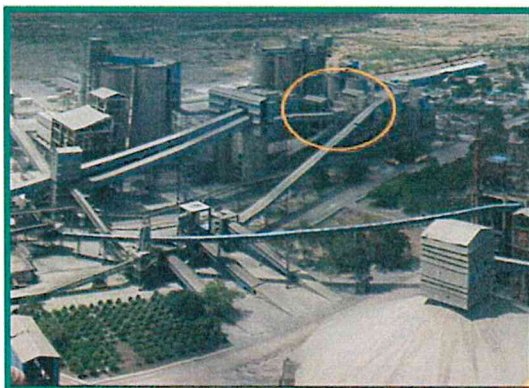
Replaced Cement Mill-2&3 ESPs by Baghouse
