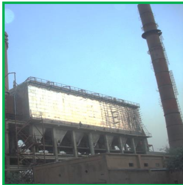
Replaced L-1 K line ESP by Baghouse
