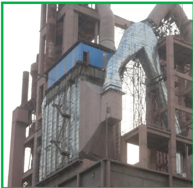
Replaced L-1 C line ESP by Baghouse
