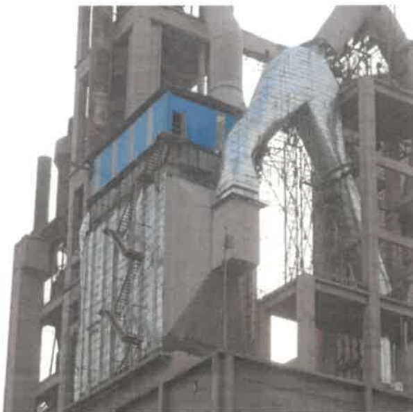
Replaced L-1 C line ESP by Baghouse
