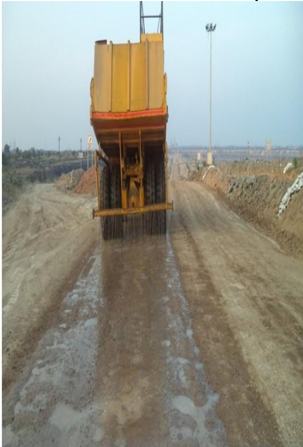
Water Sprinklers at haul road
